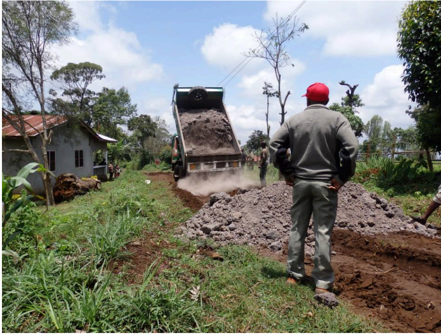
A truck unloading gravel along the Nure forest road, overseen by Mr Natai.
