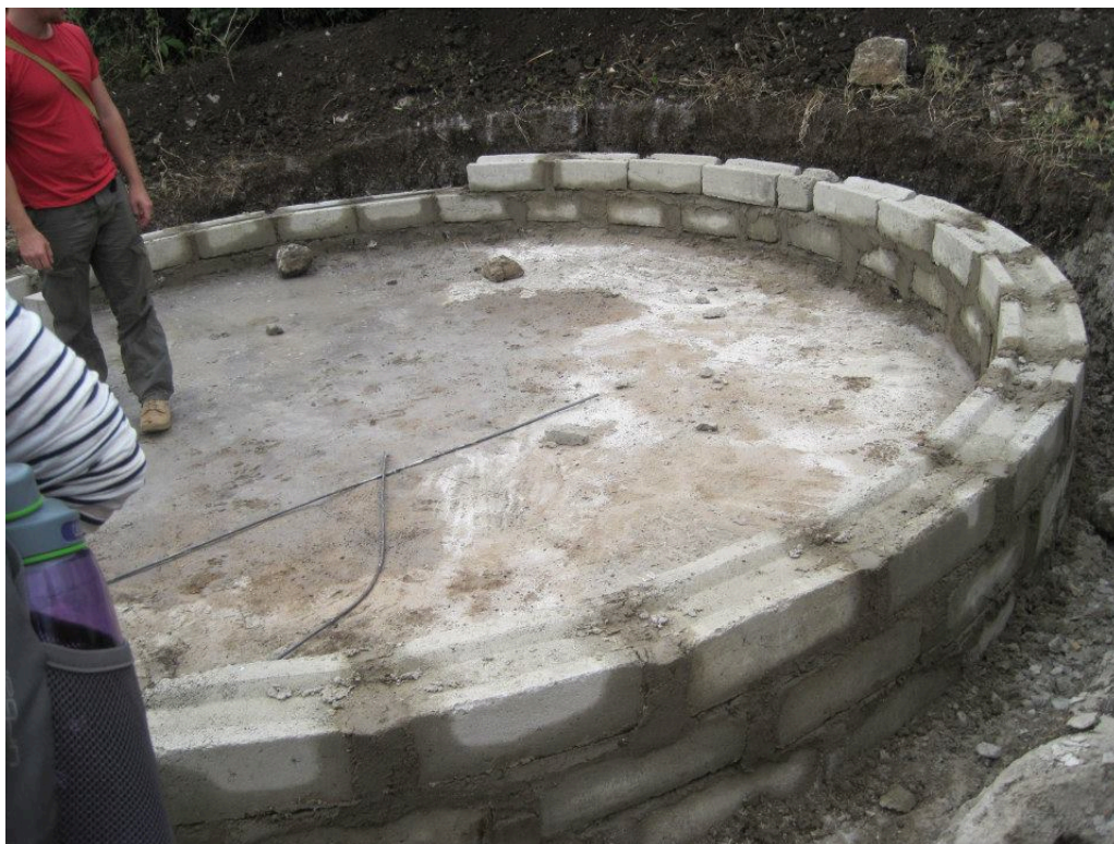
Clockwise from Top Left: concrete is spread into the foundations; rebar is laid in the second concrete layer; the walls start to take shape.
