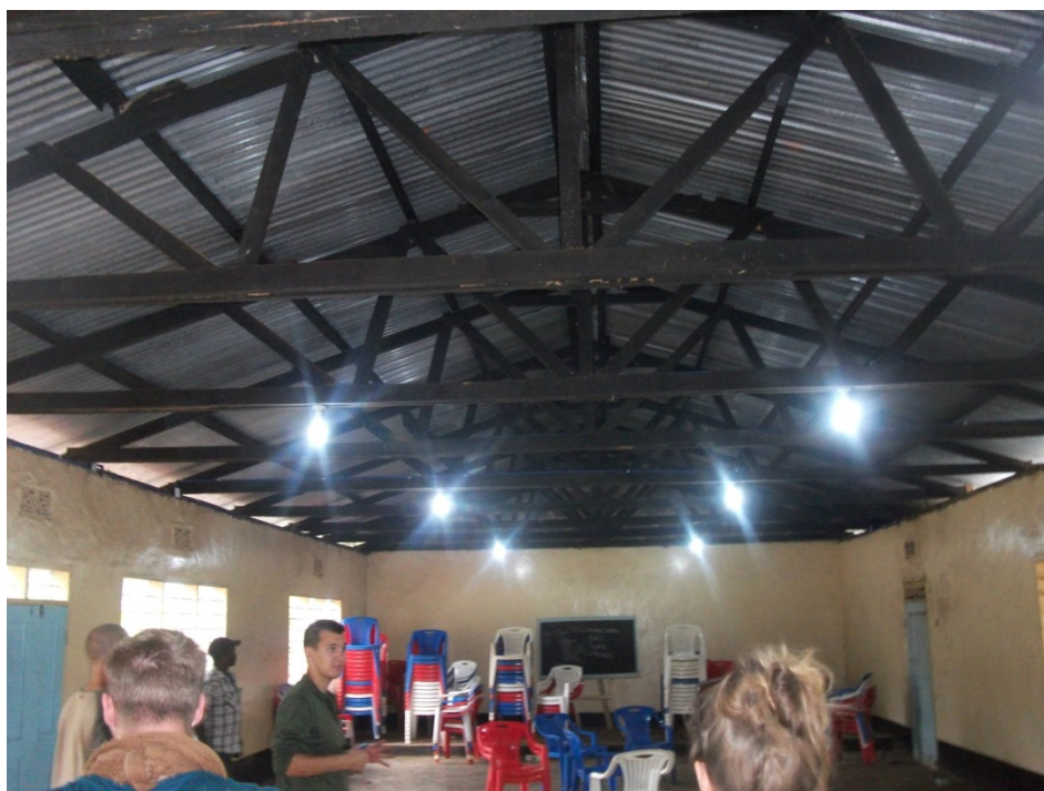
Completed- the assembly hall lit up.
