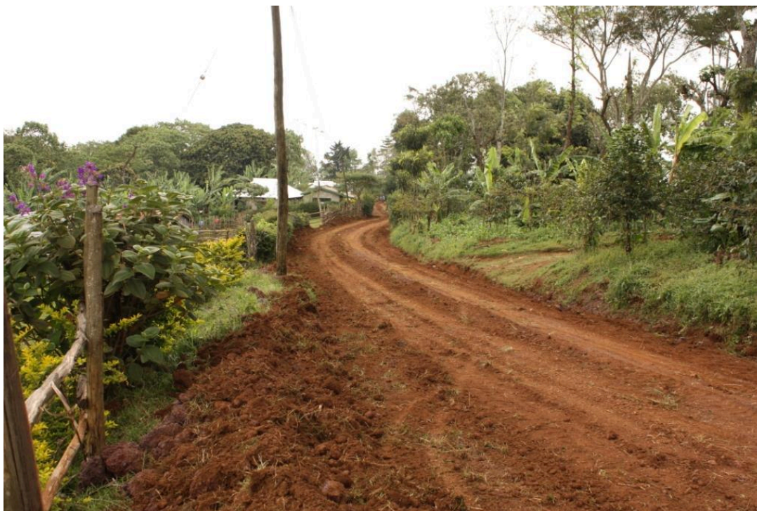
The road, after the gravel had been turned in.
