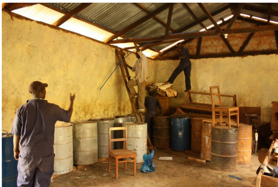
The local electrician and his team
