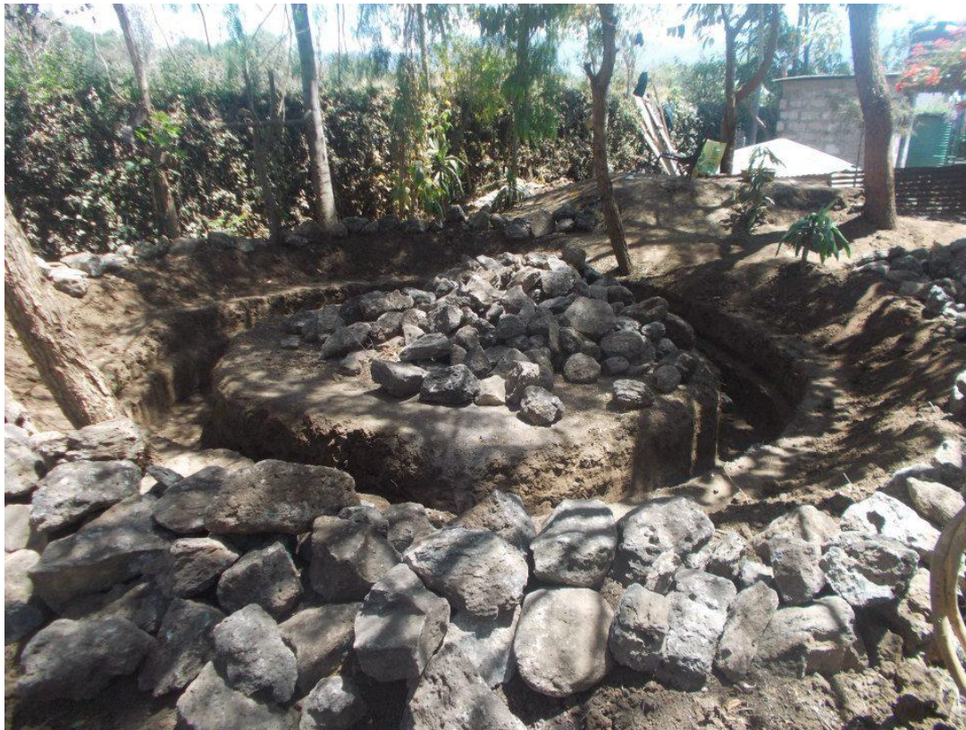
The foundations being dug, with the boulders soon to be filled in.
