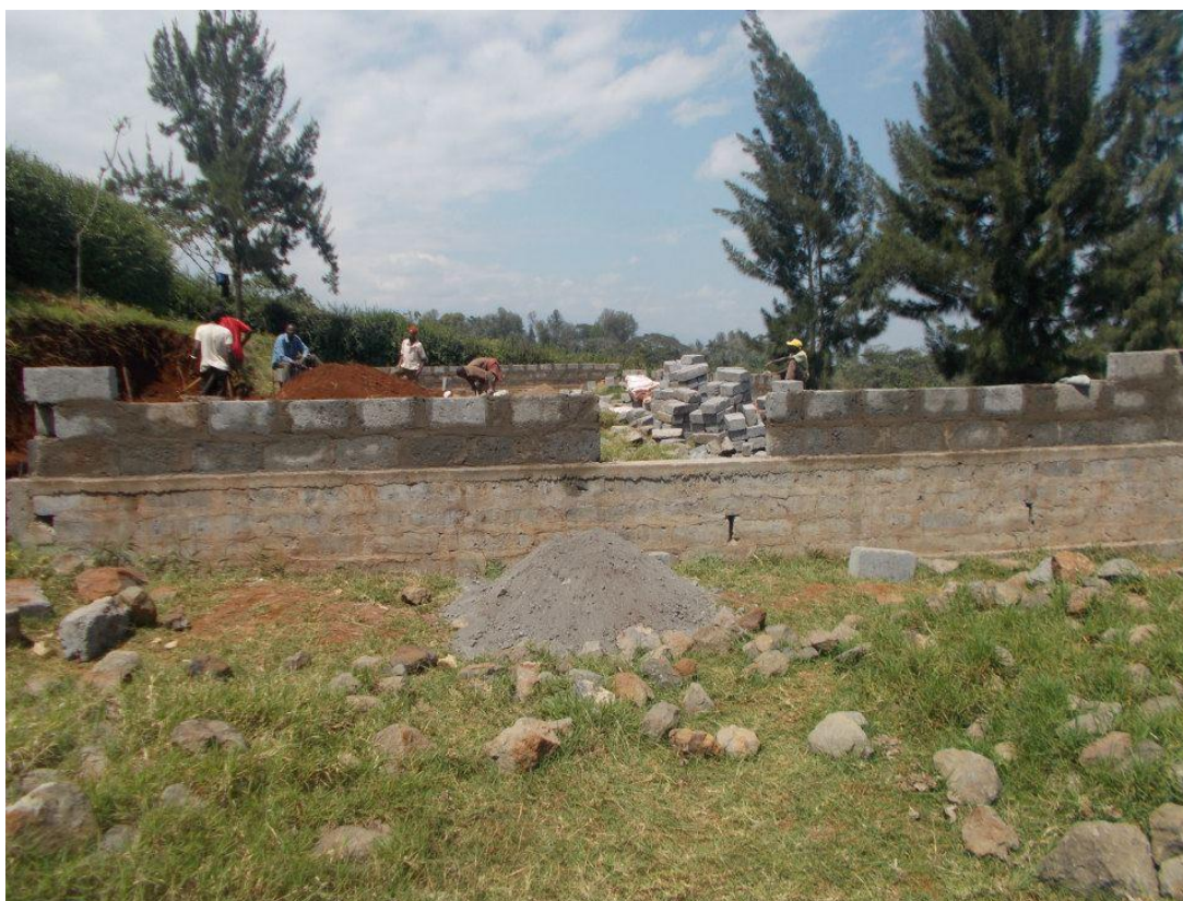
Walls of canteen starting to take shape, Nure Secondary.
