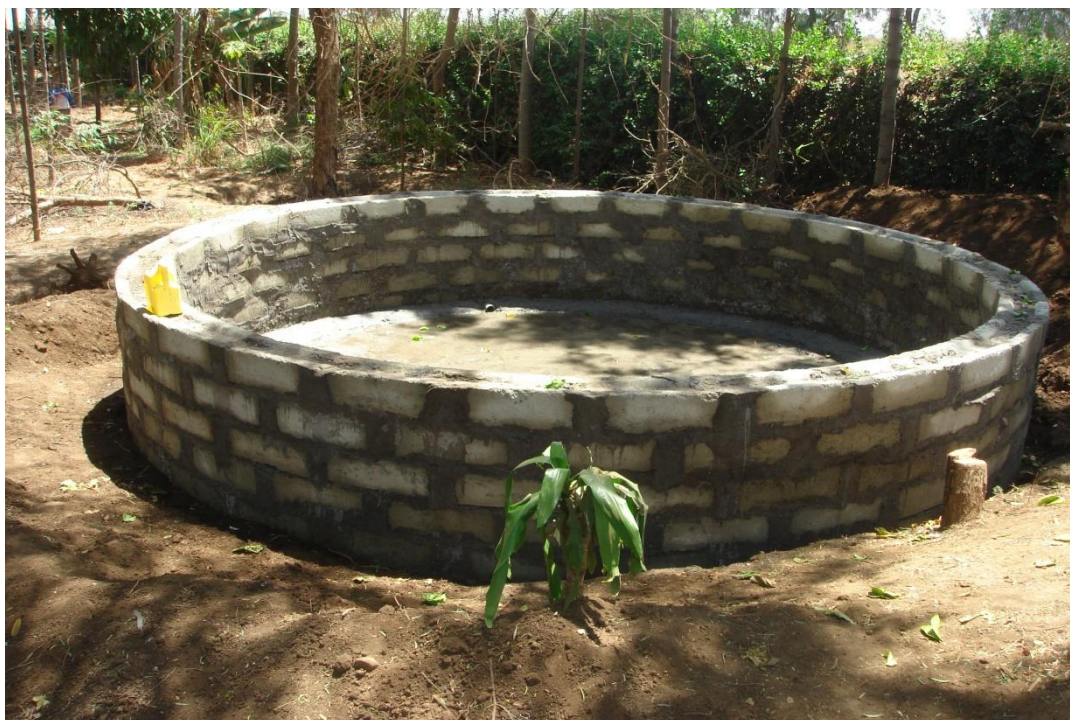
20,000 litre water tank half way to completion
