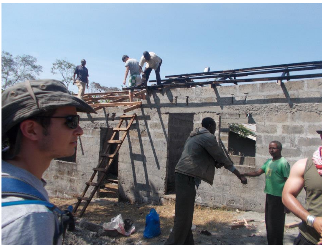
The roofing of the Dairy Co-Op though local roofers completed most of the work.
