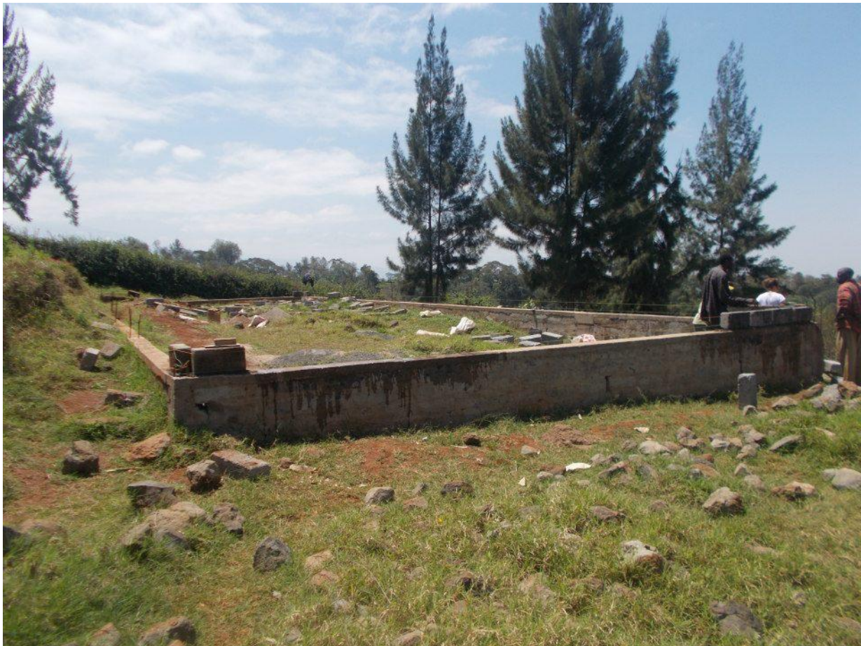
Foundations of the Assembly/Canteen hall, Nure Secondary
