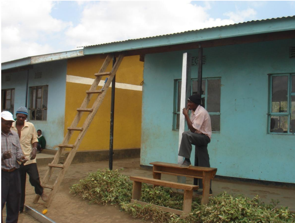
Engineers about to start work on the water harvesting gutters
